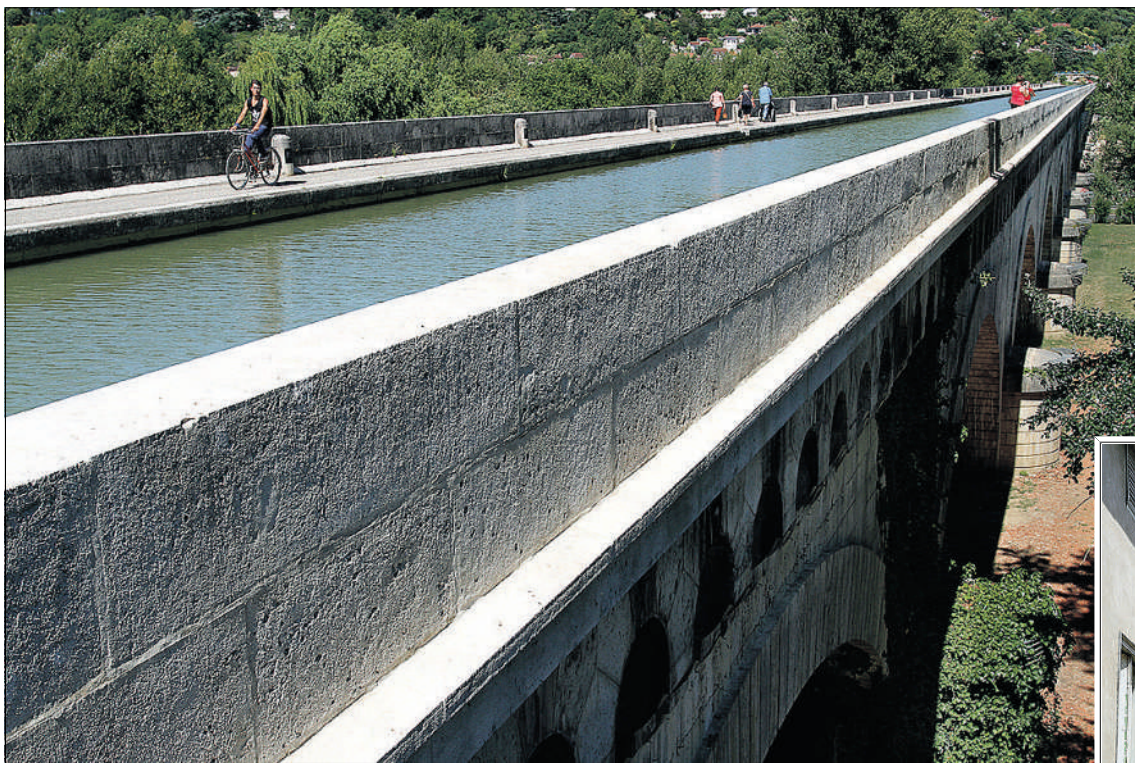
END OF THE ROAD: The picturesque viaduct canal at Agen was accompanied with a hint of sadness as our wonderful journey through Aquitaine was about to finish.
