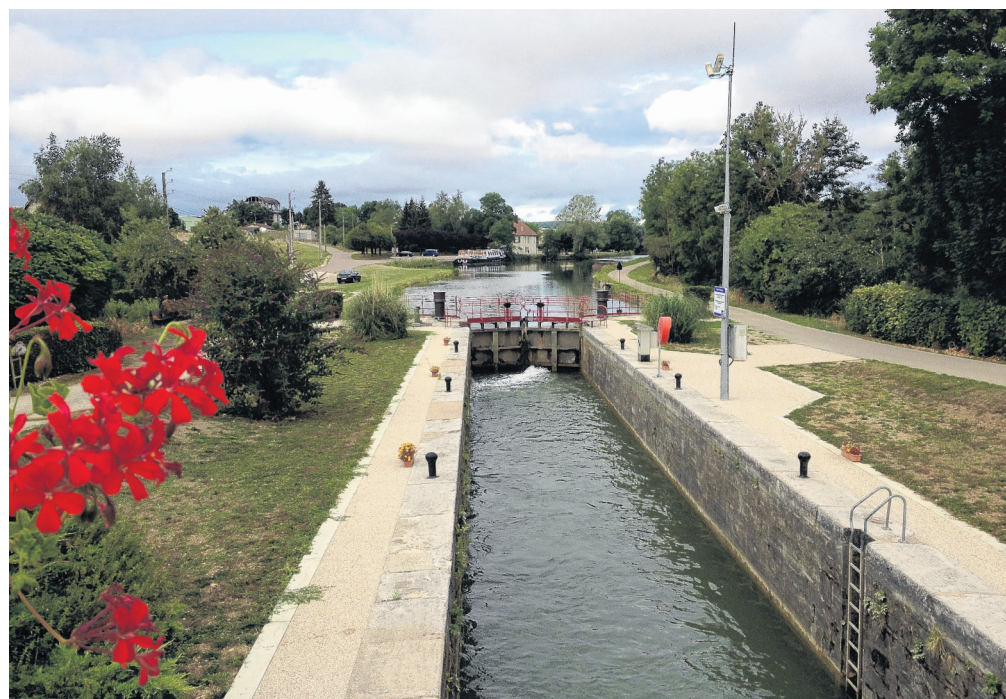
Locked in . . . Lock and towpath on the Burgundy Canal.
