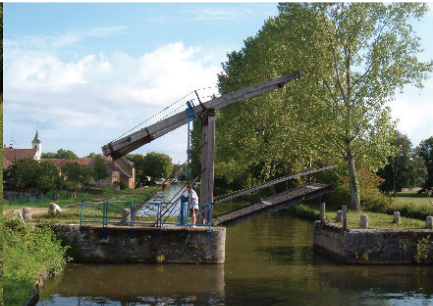
ONE OF THE FEW REMAINING WOODEN LIFT-UP BRIDGES IN FRANCE.
