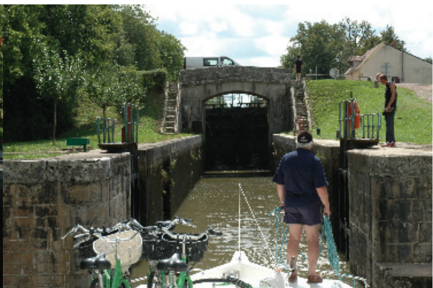
ONE OF THE FEW DOUBLE LOCKS WE ENCOUNTERED, WHICH HAS A RISE/FALL OF MORE THAN 6M.
